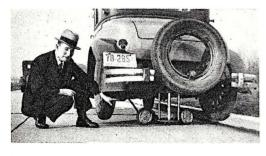
This unique car parker operates from the automobile motor. An auxiliary gear shift raises the car on the jack, swings it left or right, and lowers it into position by the curb.
