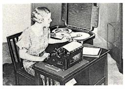
Using a magnet-sound process, this Magnetophon records sound on nerrow bands of film which can be kept on file Bands are inexpensive and resemble more costly talkie film.
