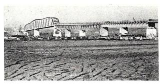
The soil shown in this picture was once the bed of the Missouri river at Onaha, Neb., but engineers wanted to build their bridge on dry land. They crowded the river into a narrow channel on one side, built half the bridge, and then pushed the river back to build the other half.
