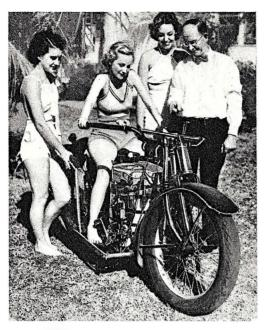
This steam driven motorcycle can average 50 miles to a gallon of fuel oil. It operates on 250 pounds of steam pressure and can run either forwards or backwards. It has no gear shift.
