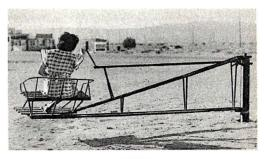
This swing can propel you 'round and 'round at a speed as high as 45 miles an hour. Motive power is obtained from gears and a crank. A brake permits free coasting.
