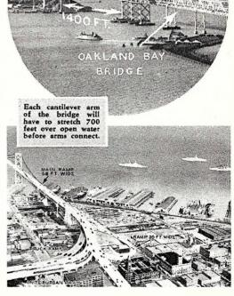
South of Market Street as it will appear in 1938. The bridge comes into San Francisco at a height of 175 feet, and the unique rampo permit traffic to flow in every wanted direction, as shown in the illustration above.
