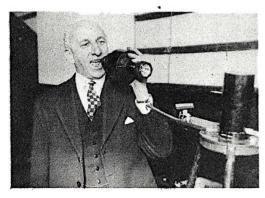
Equipped with one of these photo cell telephones you can talk to a neighbor without being connected by wires. The electric impulses travel over a light beam instead of telephone wires.
